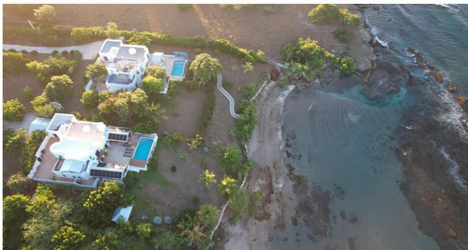
Fig 17. Section of beach between Billy's Bay and Frenchman currently only accessible by water.
